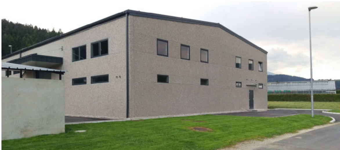
Fig. 2. Demonstration plant for soil washing technology.
