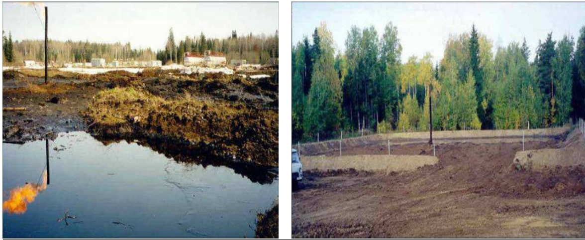
Fig. 4. Oil-contaminated site before ( left ) and after ( right ) remediation.
