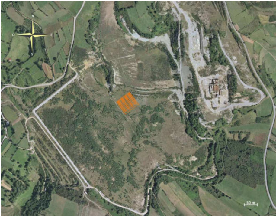
Fig. 1. View from the top on mine Rubiais in Lugo in Spain (field experiment in the center).
