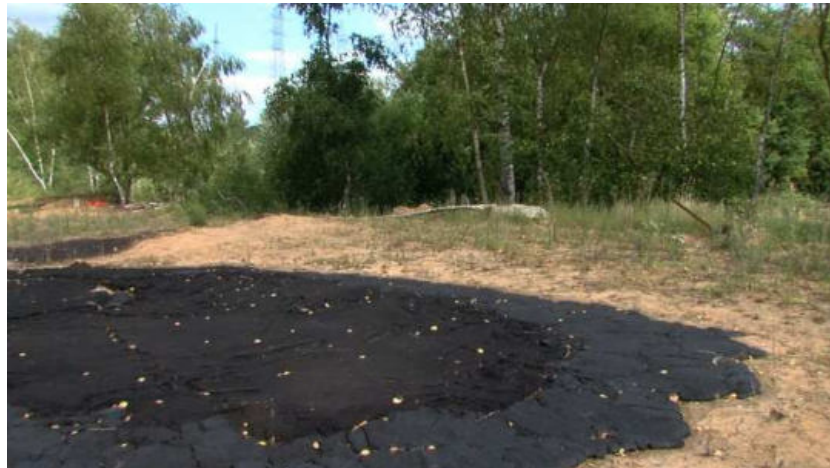
Fig. 1. Acid tar rising through covering material and spreading laterally across the surface.
